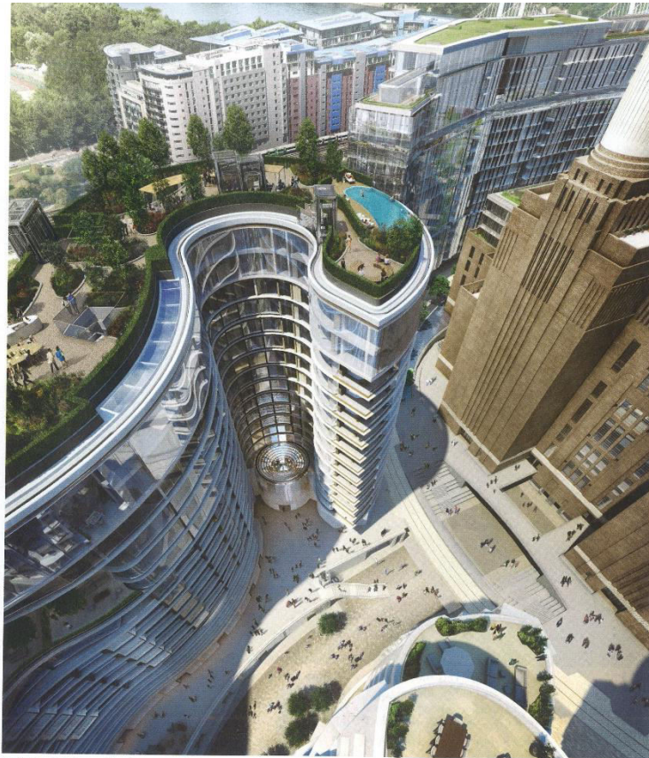
HIGH LINE Above: The reconstructed chimneys of Battersea Power Station will tower over the expansive roof gardens of the development
