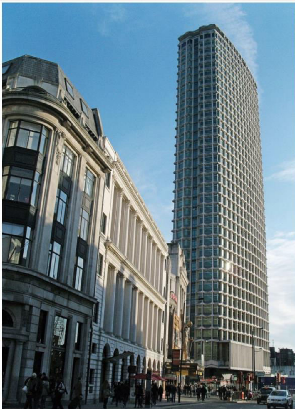
The 34-story Centre Point is the highest residential building in the West End.
