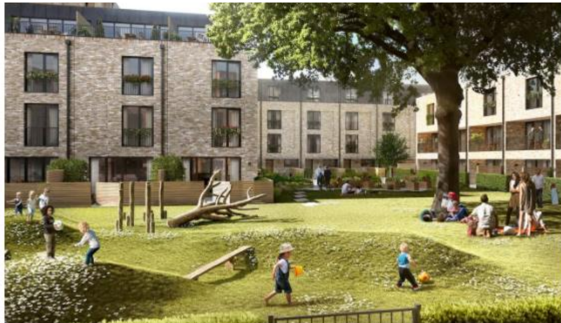
The 110 homes at Cambium are built around an 'urban meadow' with play areas
